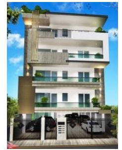
E-2135, ANSAL ESENCIA SEC-67, GURGAON 300 SQYD. ONGOING
